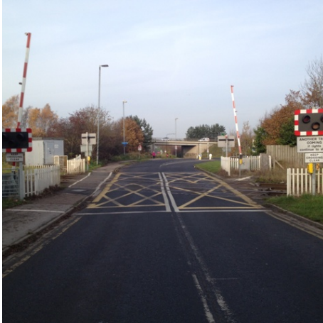
Down side crossing approach
